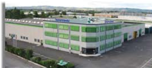
HEAD OFFICE : Via Chiesaccia, 5 - Crespellano - Bologna - ITALY
